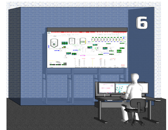
Step 6 - Commissioning of the upgraded LED video wall and closure of any gaps in the enclosure
