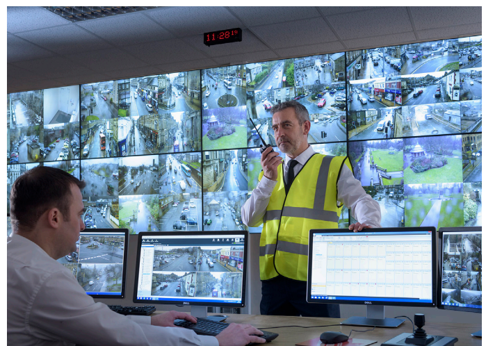
Calderdale Council CCTV Centre, UK
